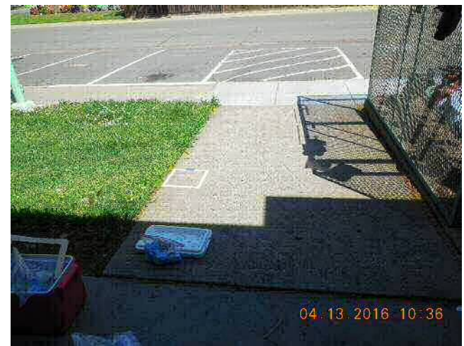
Range Building Exterior Walkway Sample 07Wipe
